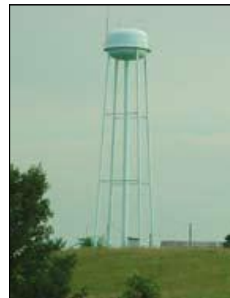
100,000 gallon Storage Tank behind Office Building on KY 259 N.
