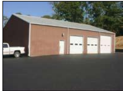
Maintenance Building located on KY 259 North.
