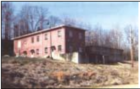
Brownsville Treatment Plant after 1 million gallon per day upgrade.
