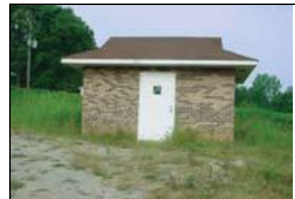
Booster Station located on KY 259 South near Fairview.
