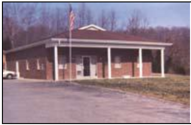
Office Building located on KY 259 North of Brownsville.
