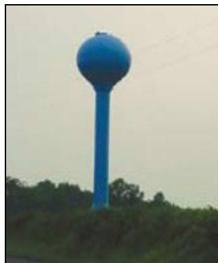
A Tank and Booster Station located at Dog Creek on KY 1015.
