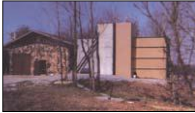
Wax Treatment Plant after upgrading to 1/2 million per day.
